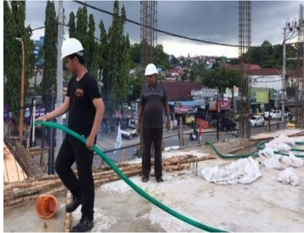
Gambar 10. Proses perawatan beton
