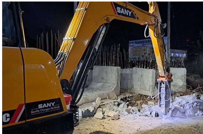
Gambar 2. Proses pembongkaran Road Crossing Segmen 1
